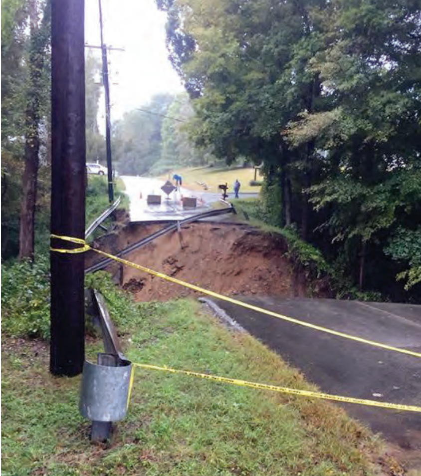
Floodwaters battered a stretch of Neptune Avenue, finally carrying it away and leaving a deep rift. Photo courtesy of Jacob Spurlock.
