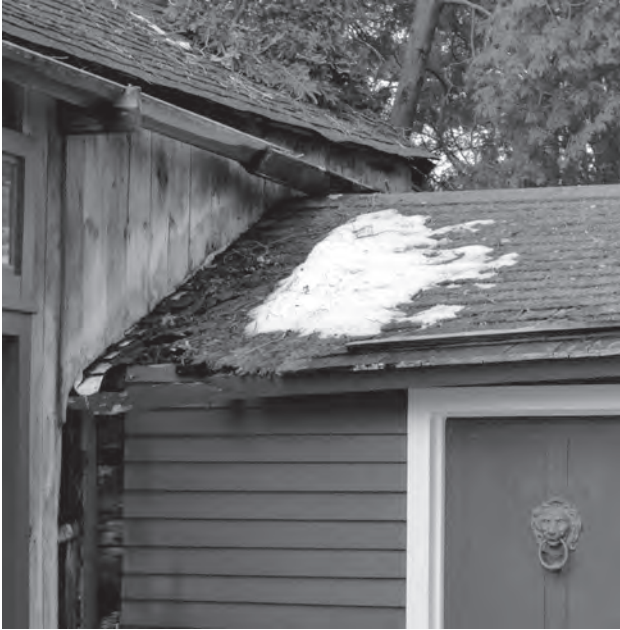
Broken gutters and holes in the roof result in leaking inside the garage area of the barn. Connecticut Landmarks, which owns the Palmer–Warner property, wants to renovate the barn for use as a visitor center, but seems to have done little work on the property in the 13 years it has had ownership. Photo by Russell Shaddox.
