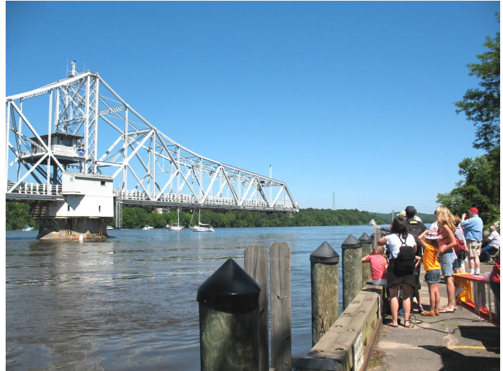
Swing Bridge Centennial, Photo by Patti Dzienis
